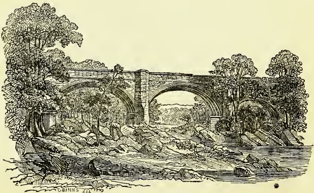
KIRKBY LONSDALE BRIDGE.—SOUTH VIEW.
